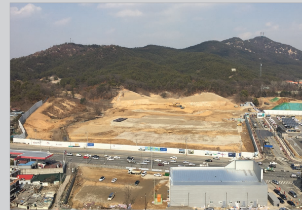
[Site preparation (March 2017)]
