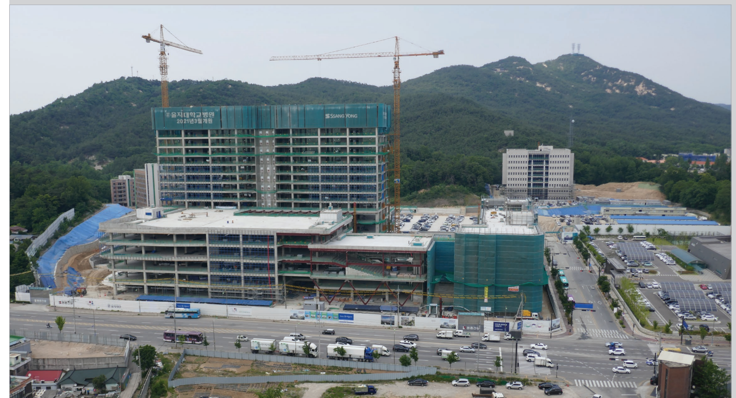
[Completion of interior, exterior and utility work (June 2019)]
