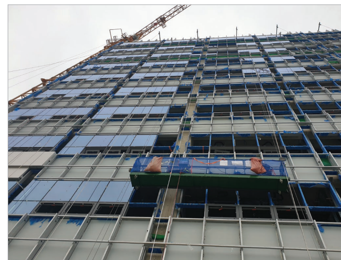
[Glass being installed on the first floor of the hospital building]
