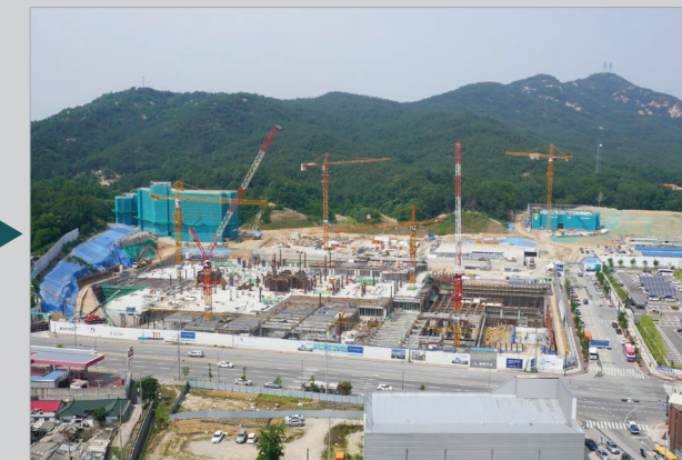
[Frame construction for the main university building (4F) (June 2018)]
