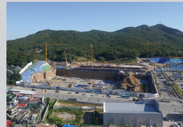
[Frame construction (September 2017)]
